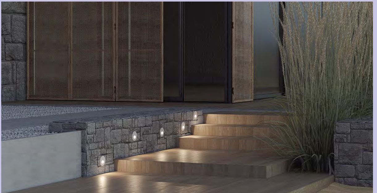
Bil Staircase Lighting
